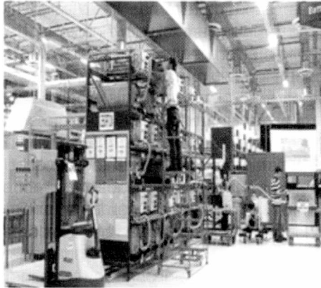
Factory 2.0: GE's advanced battery plant "Industrial Internet"
